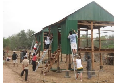
Adding floors and siding
